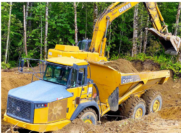
Earth overburden from the site is moved to fill a previously excavated area.
