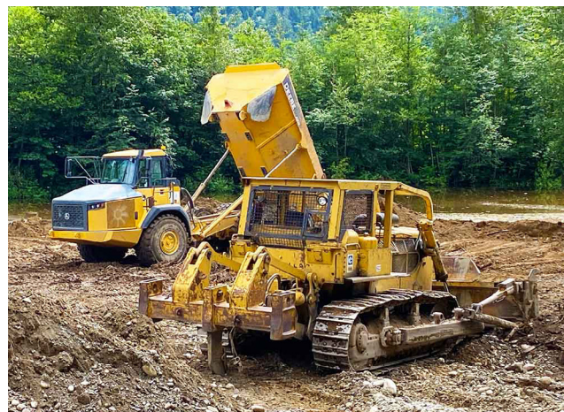
Earth overburden from the site is moved to fill a previously excavated area.
